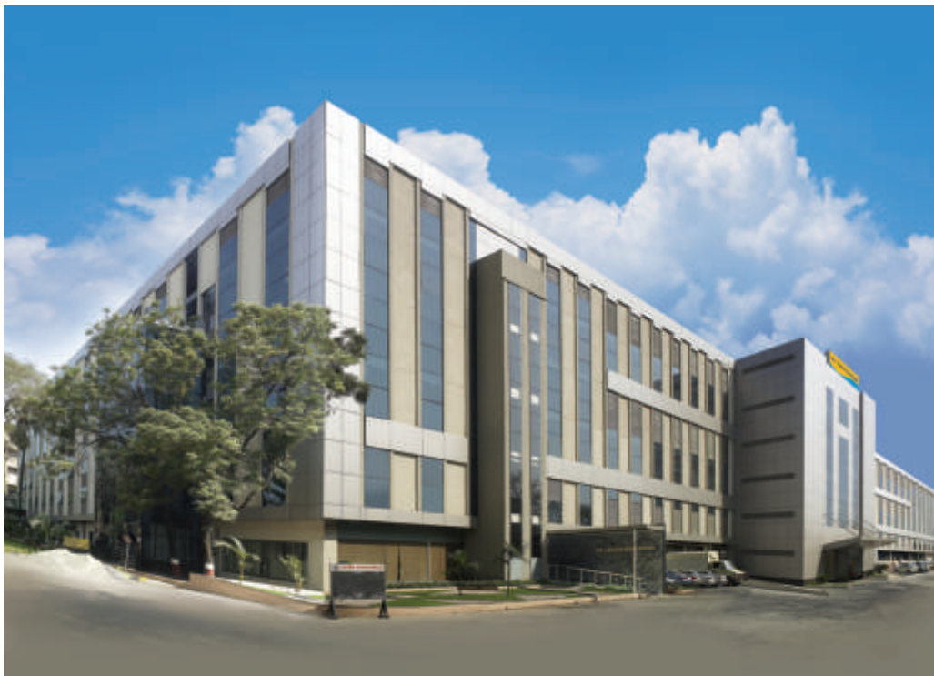
Switchgear Factory, Mumbai
